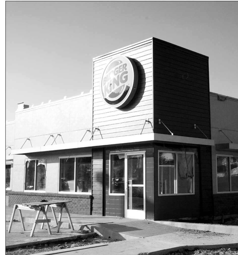
Where's the beef? Students in withdrawal during renovations. YB Lee/Staff Photographer
